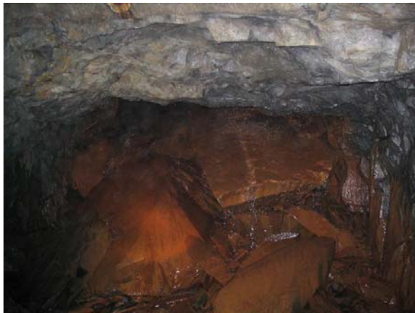
This chamber had obviously collapsed given the big size of the boulders, and water pours over them into the level.
